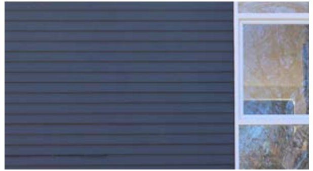
Horizontal beveled wood siding (recommended).
