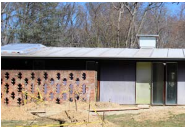
Perforated brick privacy screen and original cupola (recommended).
