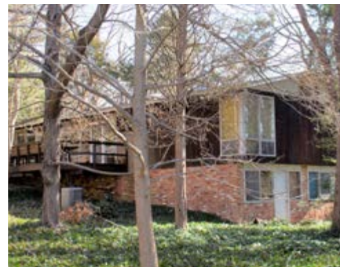
A “banked slope” building with above-ground brick walls that extend from the foundation (recommended).
