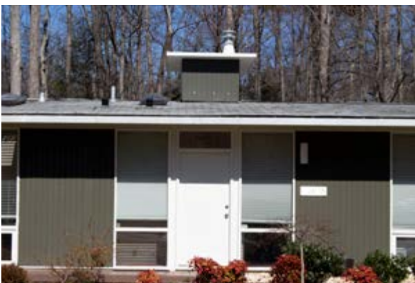
Retention of rooftop cupola for ventilation (recommended).
