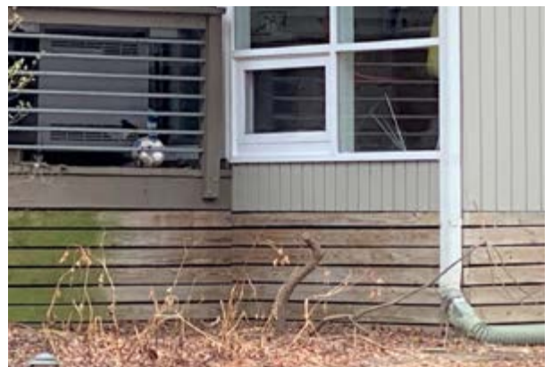
Horizontal wood cladding used as foundation veneer (not recommended).
