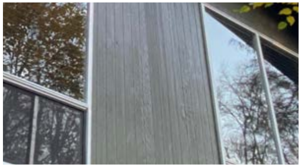
Vertical wood siding (T-111) and glazing (recommended).
