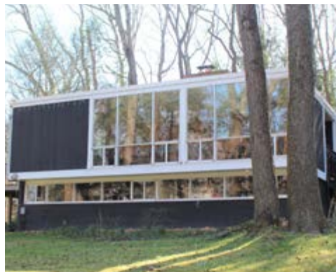
A “banked slope” building with above-ground concrete block foundation walls (recommended).
