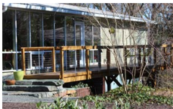
New deck with wood and cable railings (recommended).
