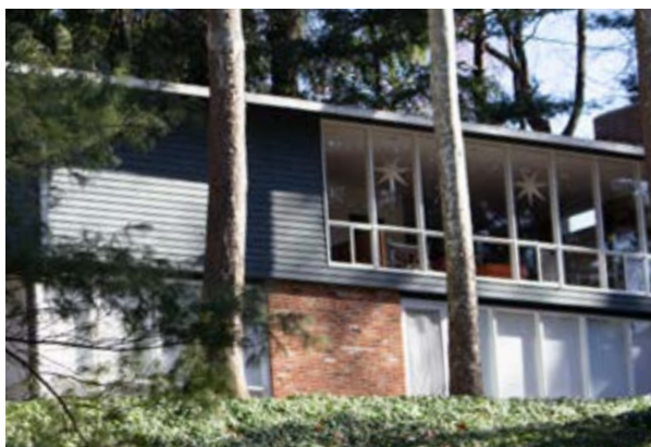
Beveled horizontal wood cladding used in combination with glazing and brick veneer (recommended).
