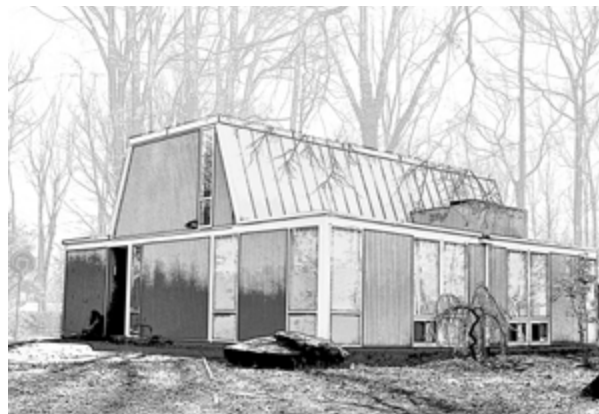
Incompatible second-story addition with an irregular roofline (not recommended).
