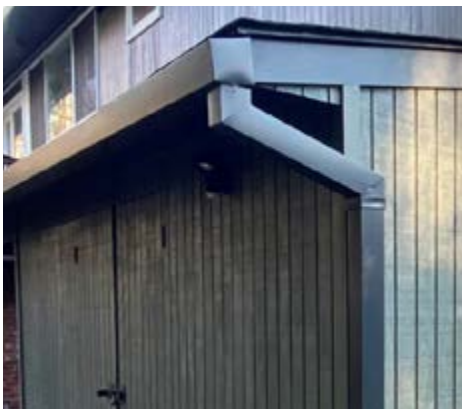
Detail of a low-profile gutter (recommended).
