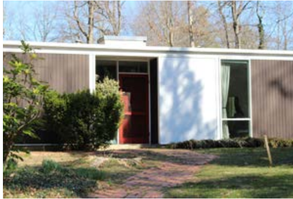
Flat roof with low cupola and no overhanging eaves (recommended).
